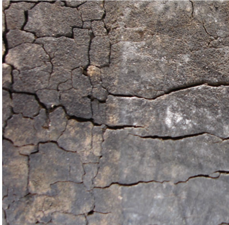
Porous surface caused by subjection to chemicals
