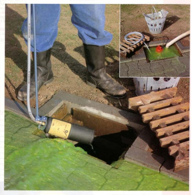
Not all the round, oval, lateral or slit-shaped gullies found around the world can be sealed with standard-type Sealing Bags to keep out pollutants after road accidents with hazardous goods. But since all gullies have a round outlet, Vetter bags seal off the outlet and use the inlet as a pump sump from which the pollutants are pumped off. A positioning rod allows the bags to be positioned correctly.
